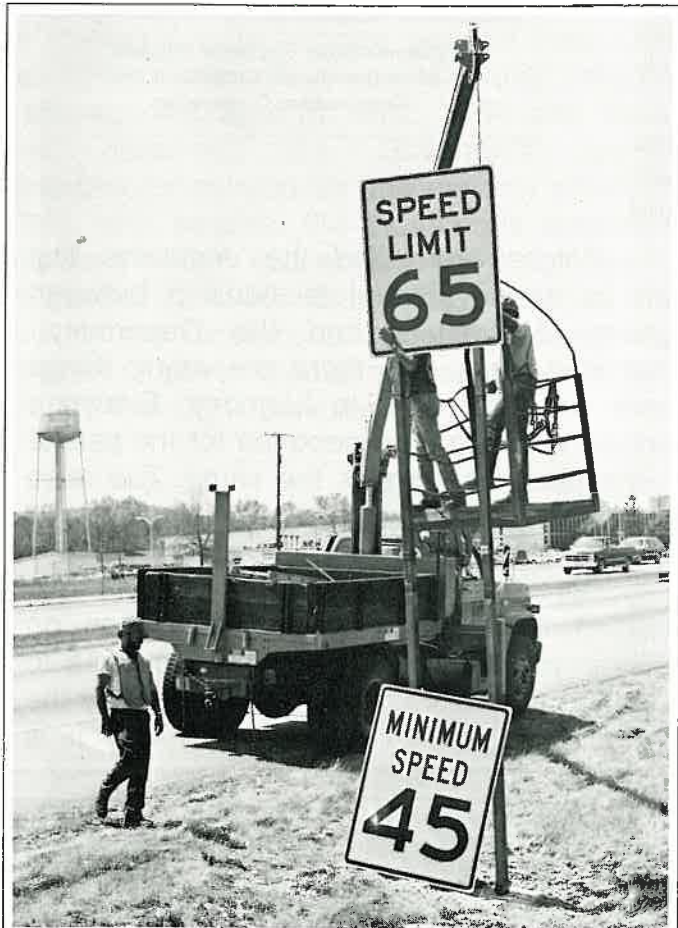
AHTD Sign Crews installed 165 new speed limit signs on the Interstate System.
